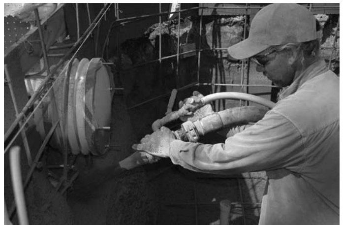
Fig. 8 BADUJET Ready for Guniting
